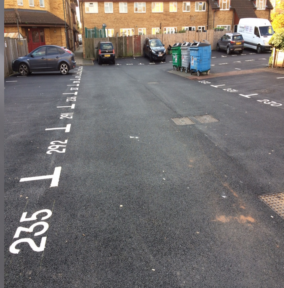
Car Park 18 After
